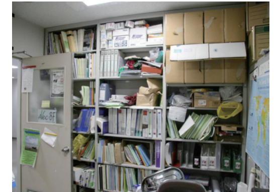
Shelves which will block the aisle when they fall (in Nagoya Univ.)
