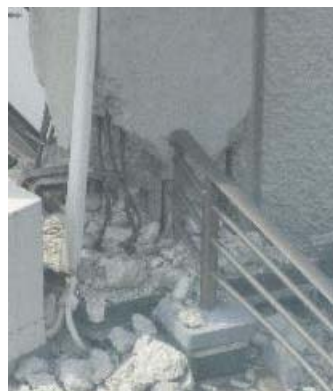
3rd-floor pillar in multi-story building demolished
