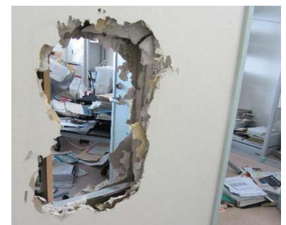
Hole pierced through a wall by rescue team as inward-opening door got stuck
