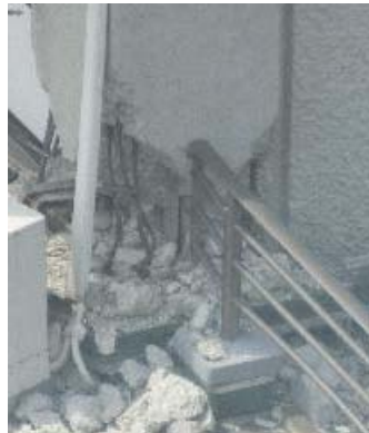
3rd-floor pillar in multi-story building demolished
